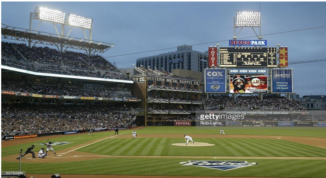
PETCO Park & Western Metal building
