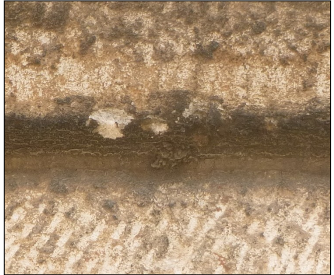
Fig. 16: Thin black crust across the relief of the decorative ripple (Ephorate of Antiquities of Athens).
