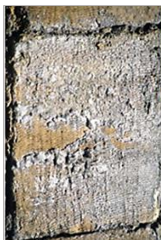
Figure 2 Salt crust formation and recrystallized on limestone (ICOMOS, 2010)
