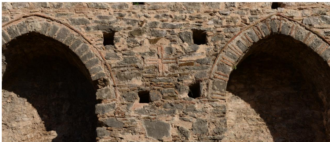
Photo 2: Decorative brickwork ornaments in the inner face of the eastern wall (personal archive)
