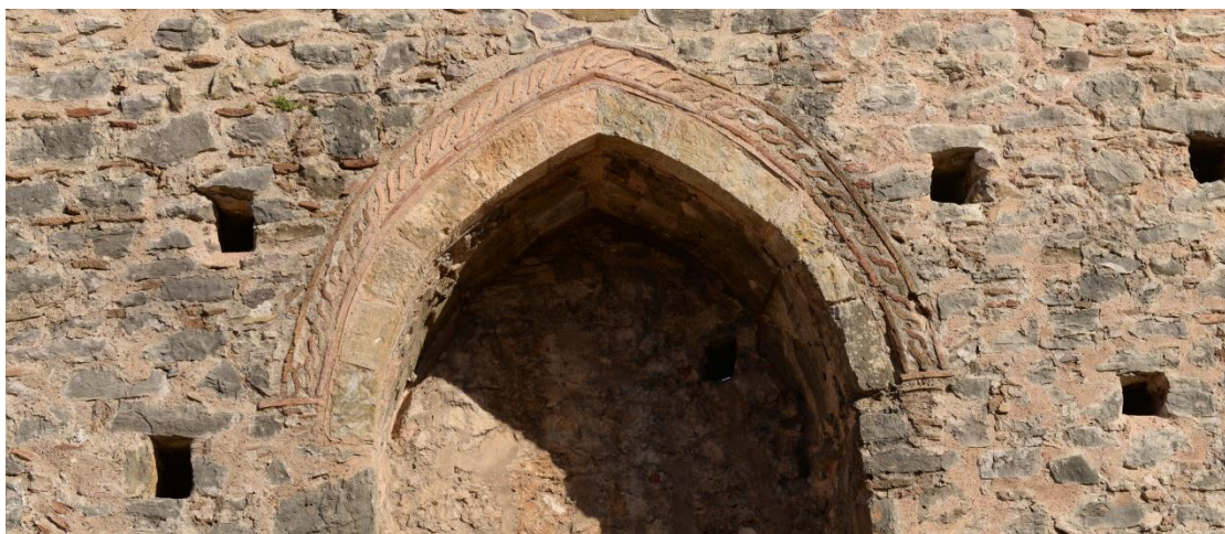
Photo 3: Relieving arch of the eastern wall with decorative brickwork (personal archive)
