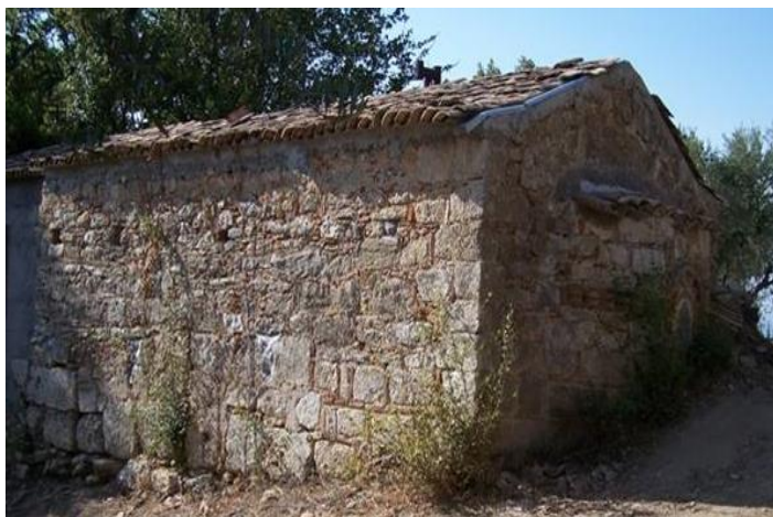
Figure 5. The little church of Panagitsa ( http://ancientthouriaexcavation.gr/images/ )
