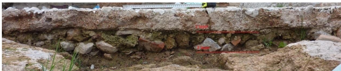
Figure 19. East side of mosaic floor B. In figure : Yellow line (a) area. Mosaic substrate with two mortar layers (Mantzana E.)
