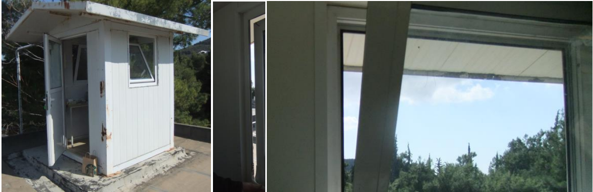
Figure 74. Left to right: Guard post with door and windows. Door and window used as ventilation openings.
