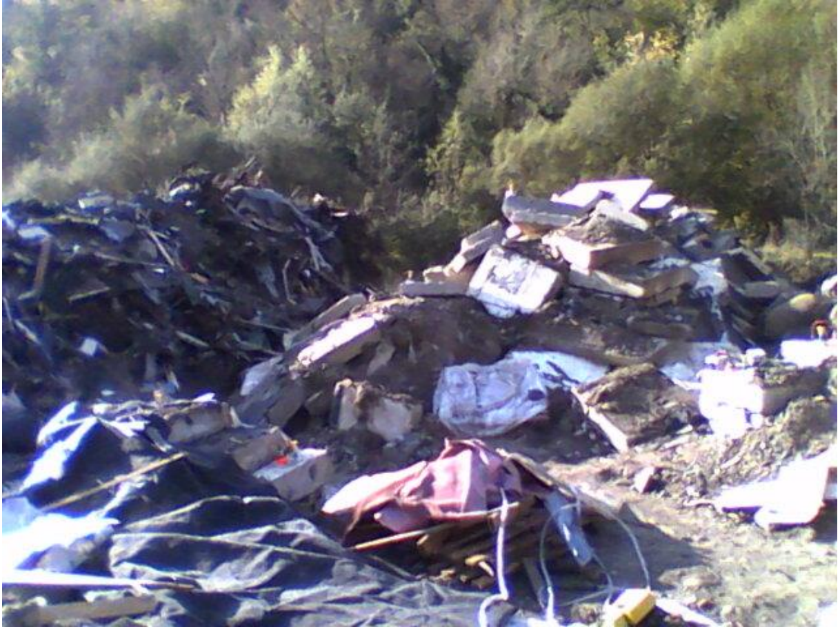
Figure 192. The test location with various rubble piles with hidden “survivors”. On the bottom right, the robotic platform is entering the rubble with a goal of reaching the area seen on the bottom left.
