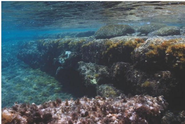
Figure 87. Underwater view of the south side of the cantilever /breakwater (Fig. Μεντόγιαννης Β. © EEA-YPPOT).
