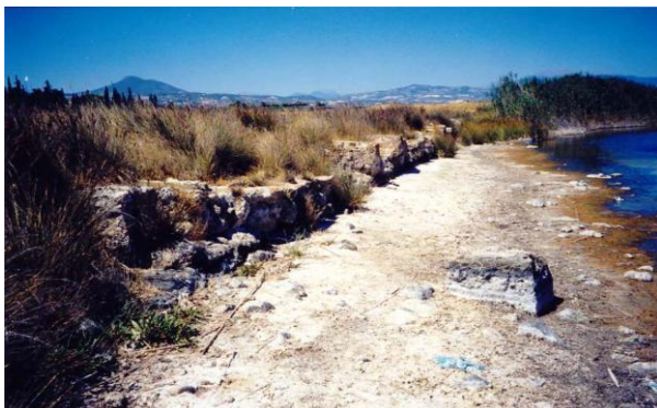
Figure 11. View of the build southern bank of the eastern basin (Θεοδούλου Θ., 2002:76, Fig. 6).
