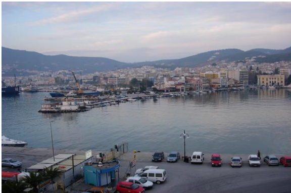
Figure 82. View of the breakwater Lantern which coincides with the s/n breakwater of the ancient southern basin
